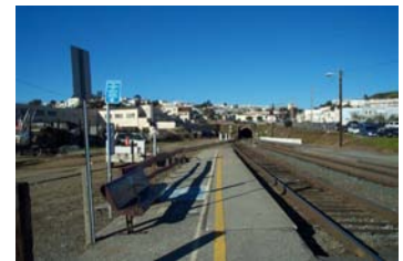
Existing Caltrain Station photo: EDAW
